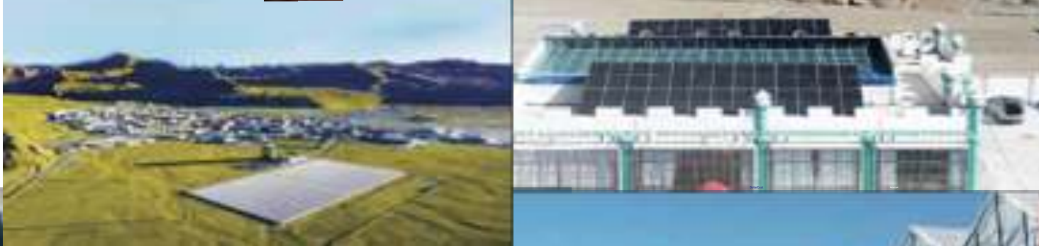
PV Solar Thermal+Energy Storage Project, Tibet
